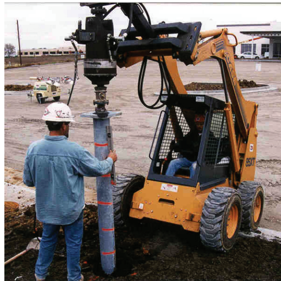
Foundation Lighting and Signs® Products are Easily Installed Using Common Construction Equipment. Figure 10-3
